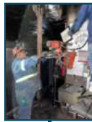
Removal of concrete cores and steel shafts
